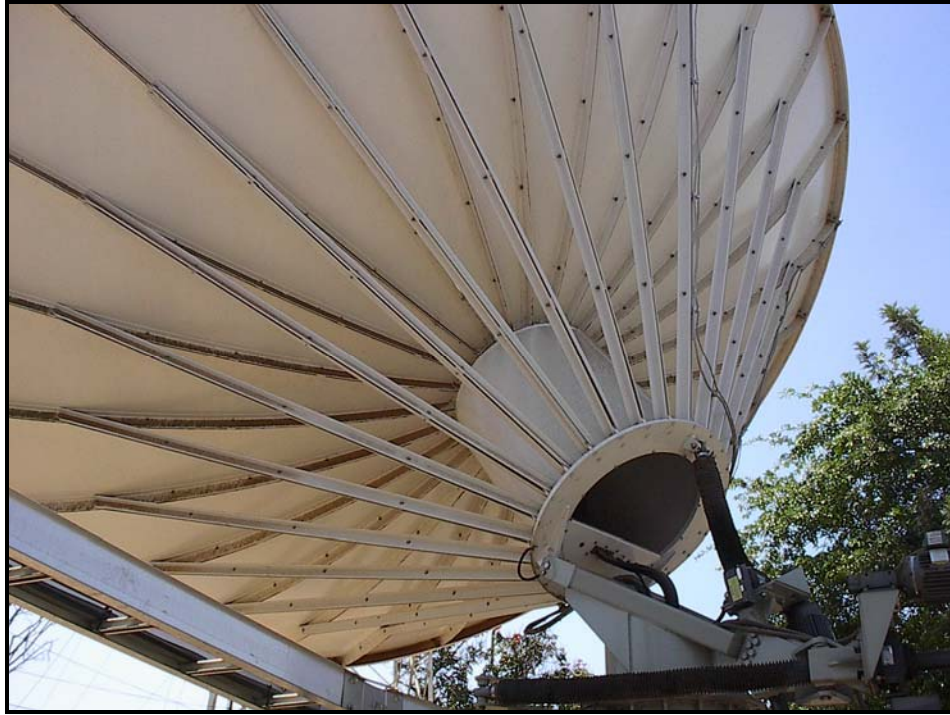
Fig 6: 9.3m antenna installation at uplink site in Kampala
