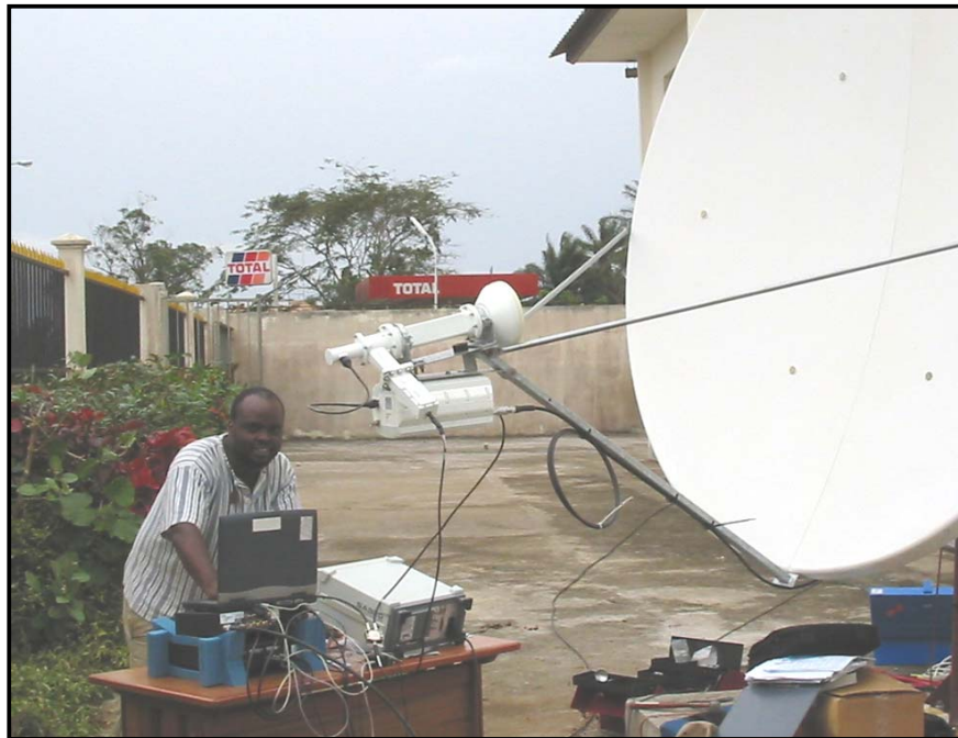
Fig 2: Commissioning VSAT station at Oyem - Gabon
