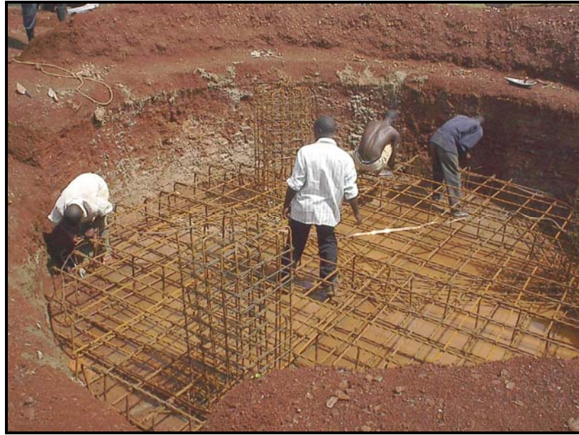
Fig 3: Tower base construction
