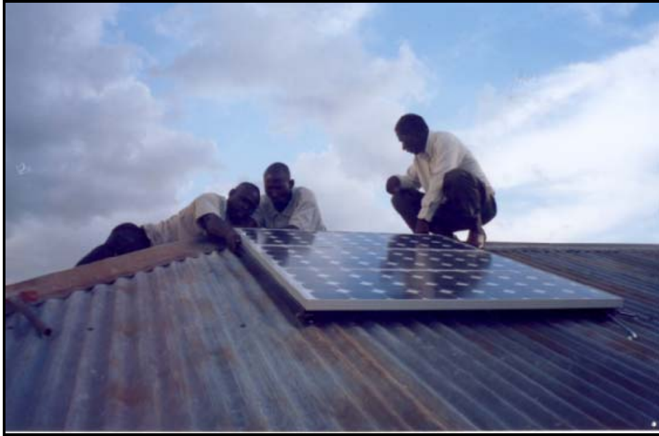
Fig 1: Installing Solar panels at Kenshunga Sub-county, Mbarara
